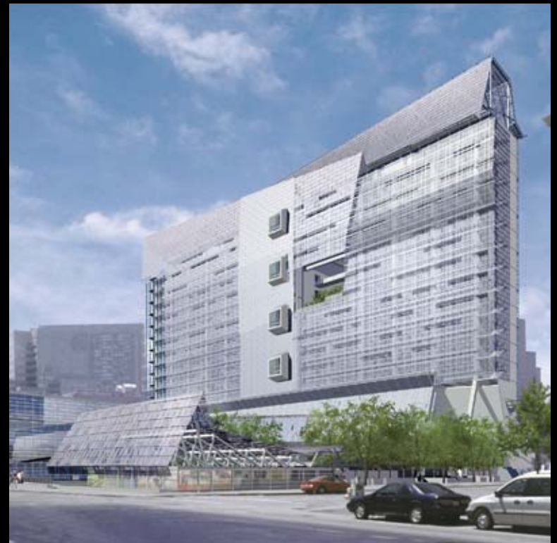
Federal Building San Francisco, CA
